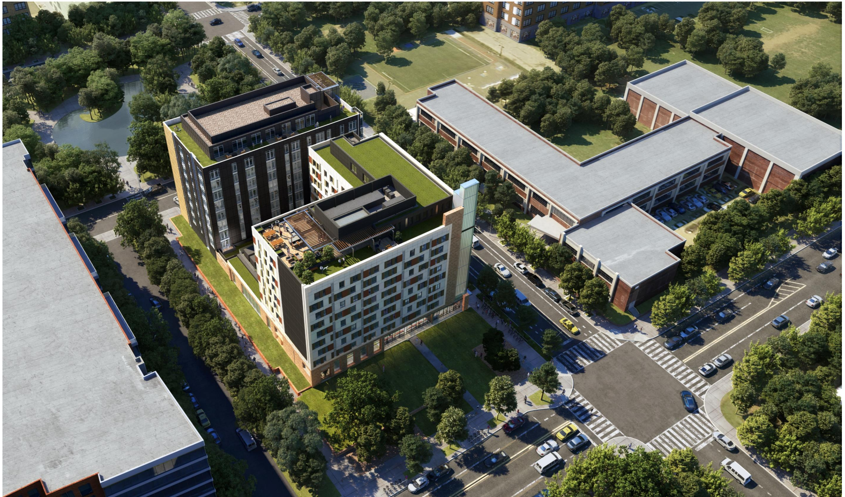
SOUTH EAST AERIAL VIEW OF SITE VIEW 4
