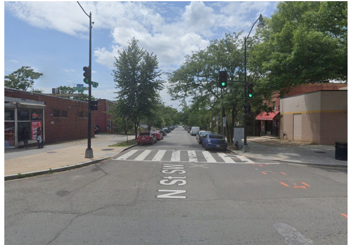
N STREET LOOKING WEST
